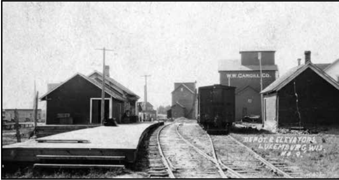
The Cargill elevator built in the 1890s in Luxemburg, Wisconsin on the Kewaunee line.
